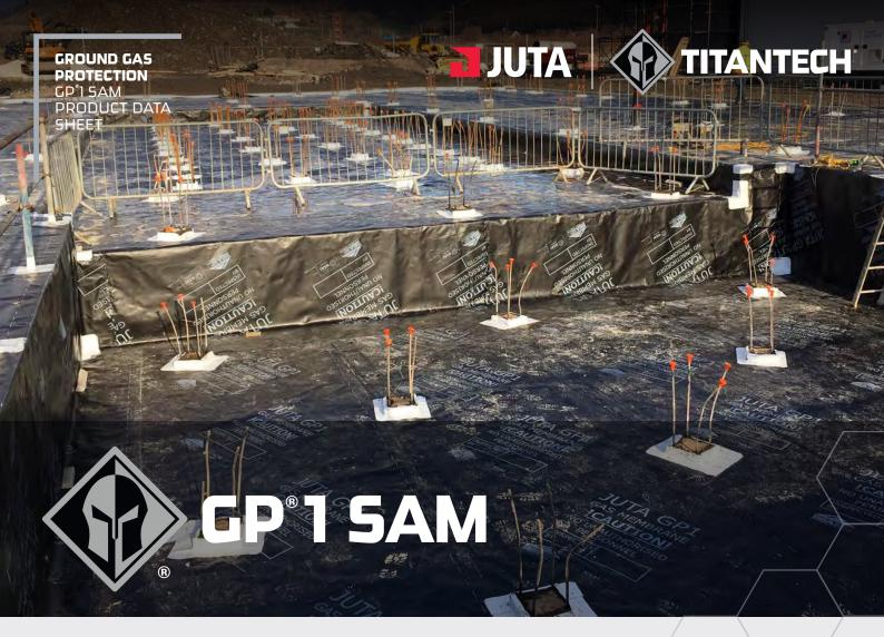
GP®1 SAM, the gas protection self adhesive membrane, is a bituminous gas proof and water proof sheet, composed of self-adhesive SBS polymer modified bitumen incorporating GP® 1 with an upper surface finish of black reinforced LDPE, and a lower surface finish of siliconized release film.
