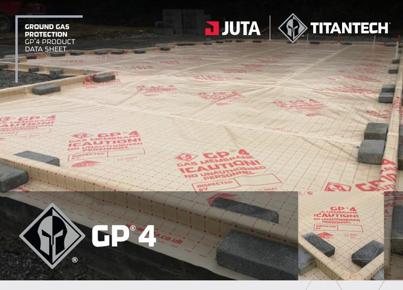
GP®4 gas barrier is a multi-layer, low density polyethylene membrane, reinforced with a polypropylene reinforcing grid. GP®4 is specifically designed and manufactured to perform as a radon, air & moisture protection system, as well as low level protection to carbon dioxide, and methane.
