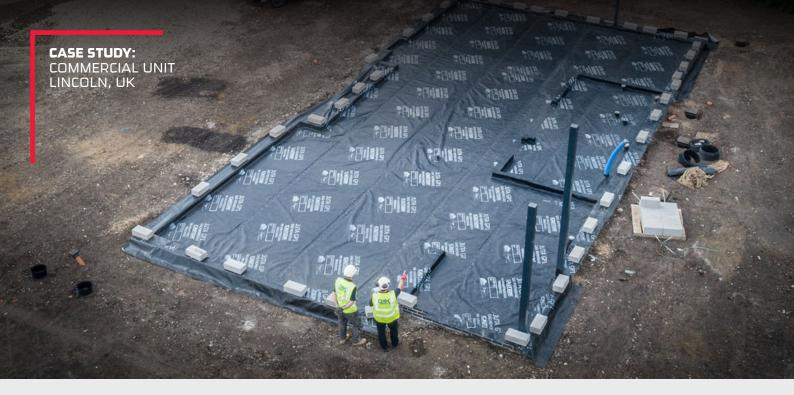
Preparation is key when installing proprietary gas membrane, to both avoid damage occurring during the installation and avoid delays when independent verifiers check the installation according to CIRIA C735.
